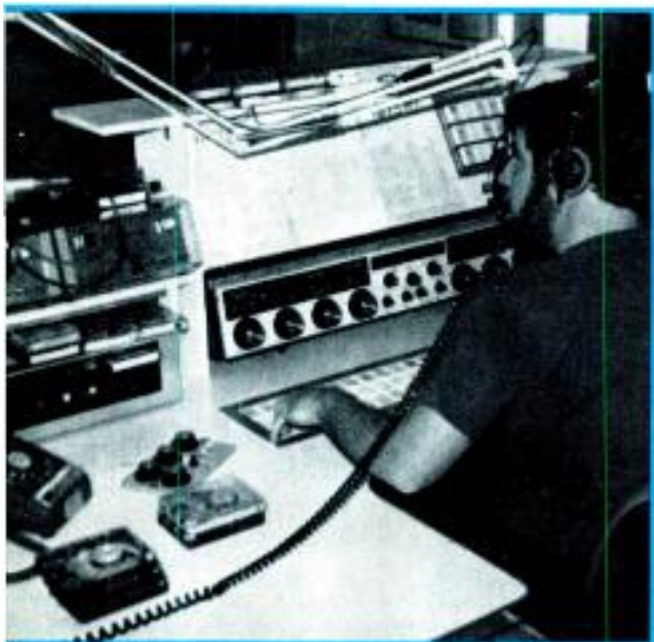
Equipment layout at KRED-AM. Source machines are arranged to be within arm's length of the operator.
